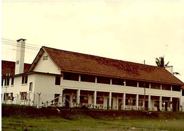
Figure 60: Block 89 at Canberra Road. Source: Sree Narayana Mission.
