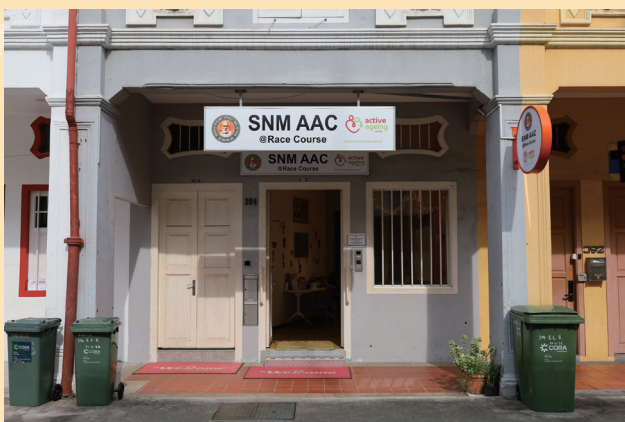
Front View of SNM AAC@Race Course at 394 Race Course Road
